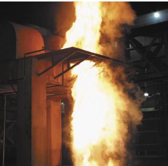
**P**ut it under pressure and confine it within piping, seals or removable-opening covers. Then, provide an available "hot" surface—hot enough to ignite mineral oil...nearby steam piping or a turbine casing will do the job. Now, wait until a flange leaks, a pipe breaks, a seal fails or a cover is left off an opening—and you have a "recipe" for one of the largest fires you could ever imagine. And, if the oil is released in a spray, it could be even larger.
