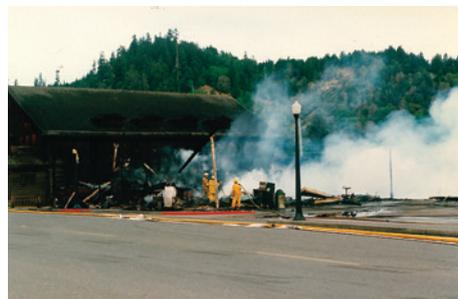
*This post-earthquake fire grew uncontrolled when damage to underground piping impaired the sprinkler system and delayed water delivery. Photo courtesy of ABS Consulting — EQE Structural Engineers Division.*
