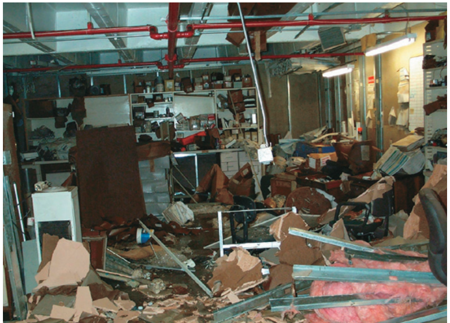
This maintenance office, located in a below-grade area, was completely submerged. Valuable maintenance records, service agreements and other articles were lost.
